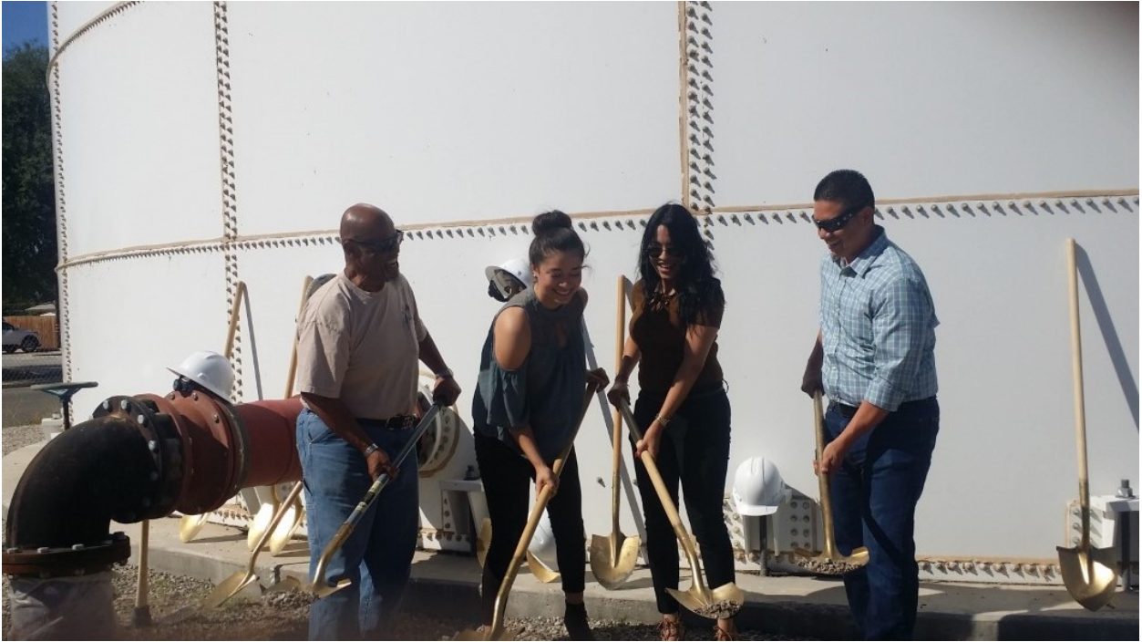
Seeley County Water District Water Treatment Plant- TTHM Improvement Project. Community Facility Program/ Water and Environmental Program Specialists.
