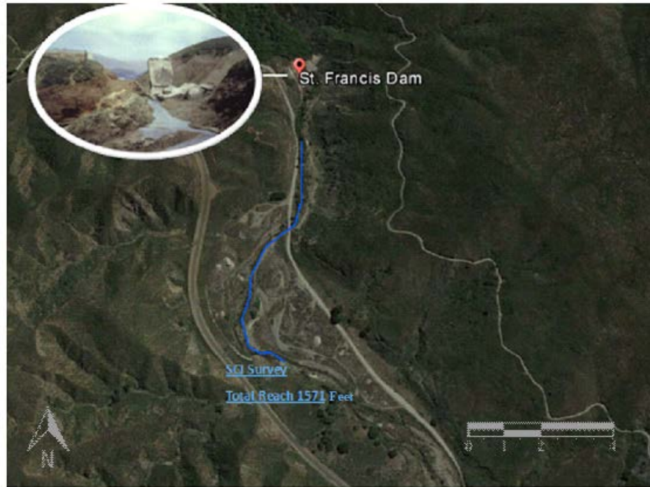
Figure 1: Study Site--Downstream of St. Francis Dam, CA
