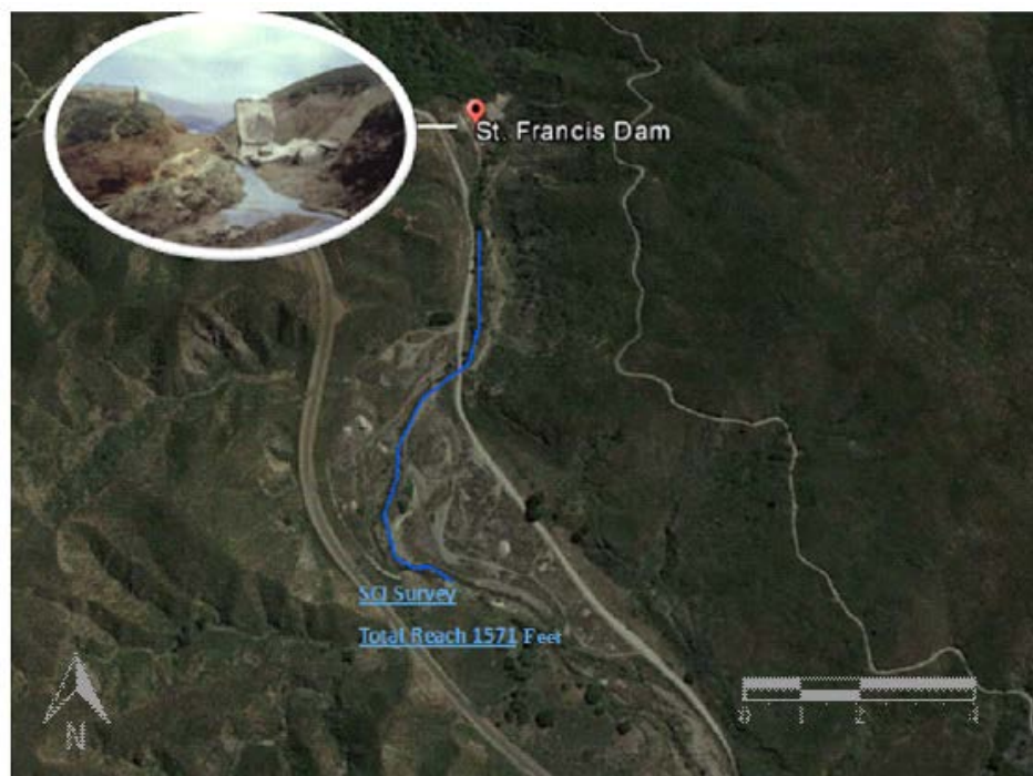
Figure 1: Study Site--Downstream of St. Francis Dam, CA
